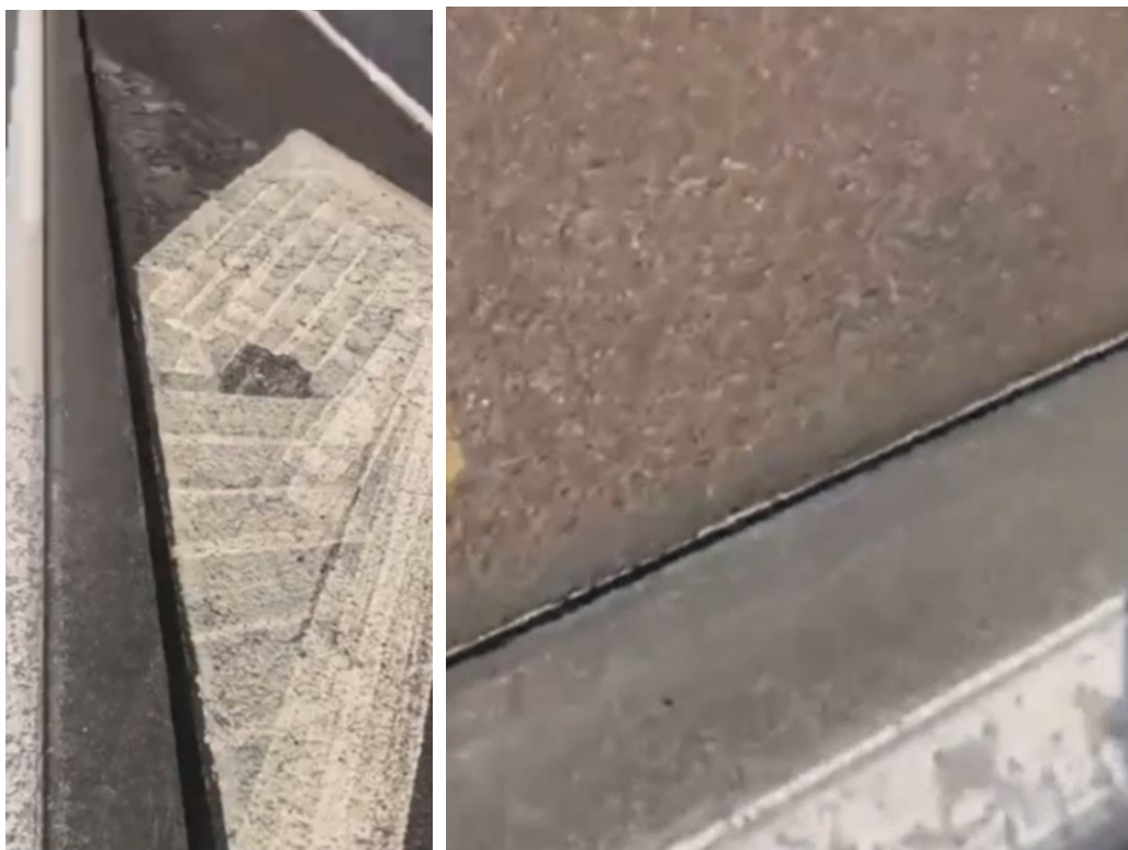
Figure 12 a \pm 50\text{mm} gap opening (left) and closing (right) on longitudinal joint between clip-on and main span. OIA 12397
