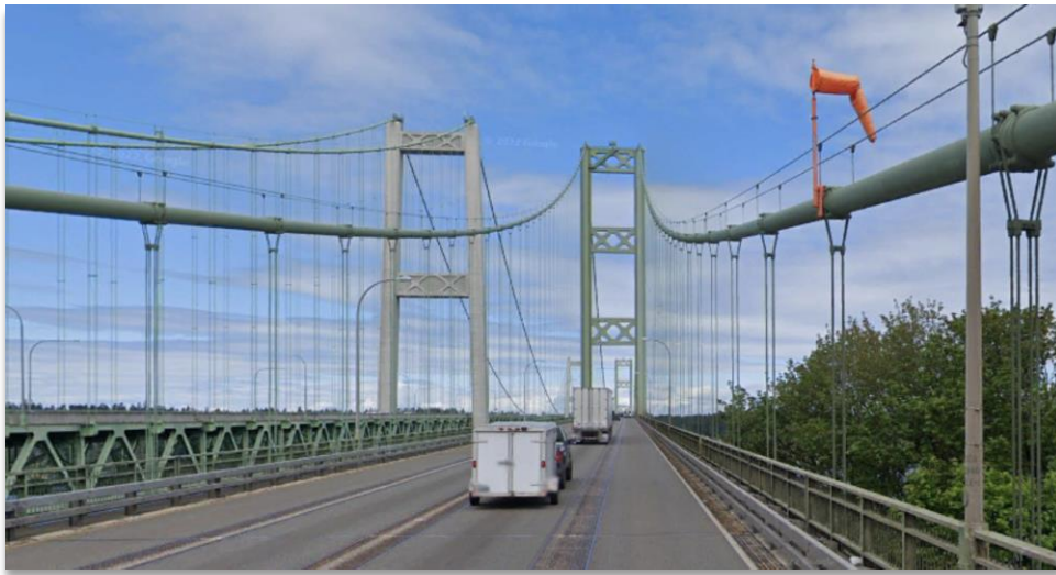
Figure 28 Windsock deployment to provide regular users with direction and strength information (Tacoma Narrow Bridge, Washington State, USA)
